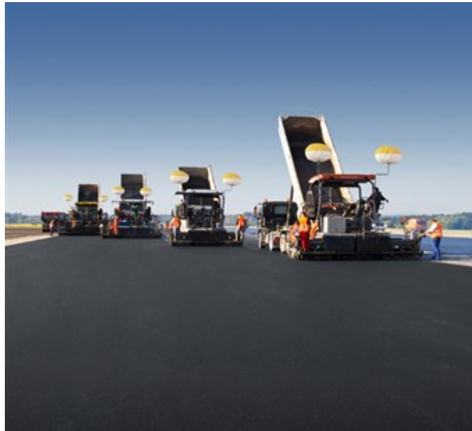
Figure 6: Echelon paving [worldhighways.com, 2011]
